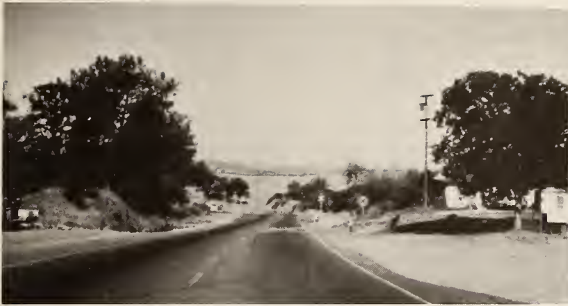
Figure 55 Driver View - 600 Feet (183m) (Amador Central Crossing)
